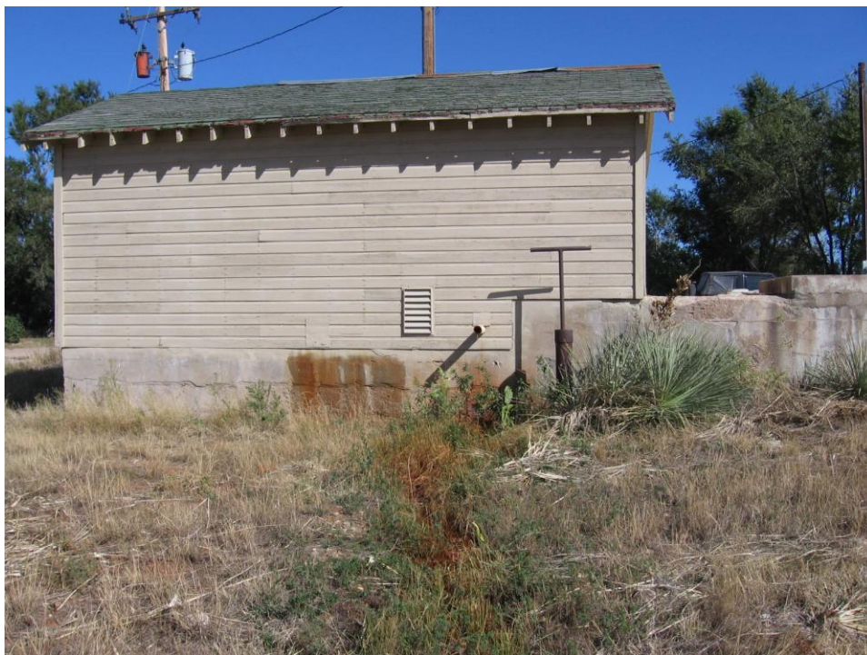
Figure 5-2. Picture of a CO-RADS System's Discharge of Spent Filter Backwash to the Ground
