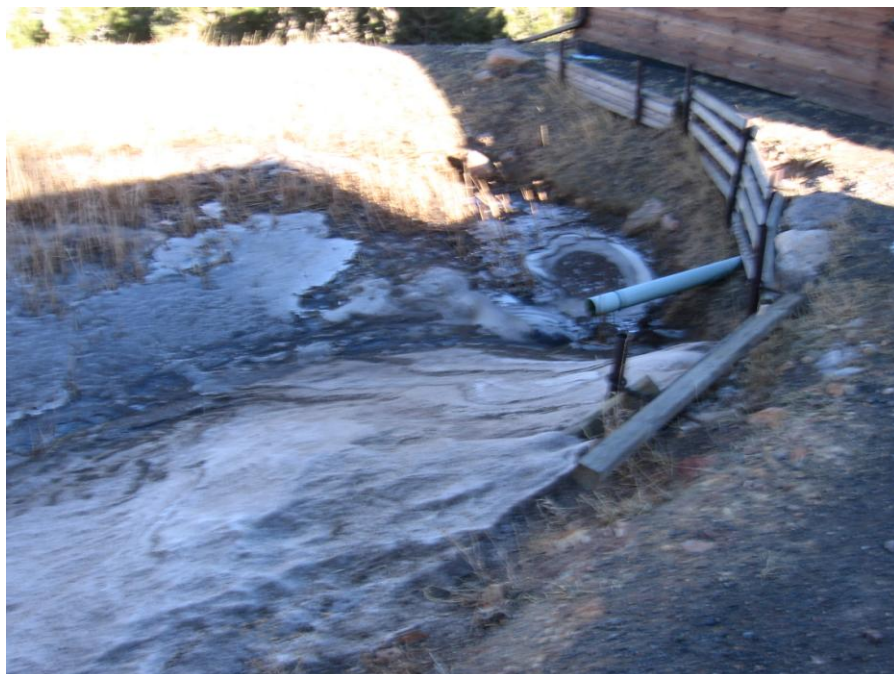
Figure 5-1. Evaporation Basin where Liquid Residuals from Radionuclide Treatment are Discharged at one of the CO-RADS Systems
